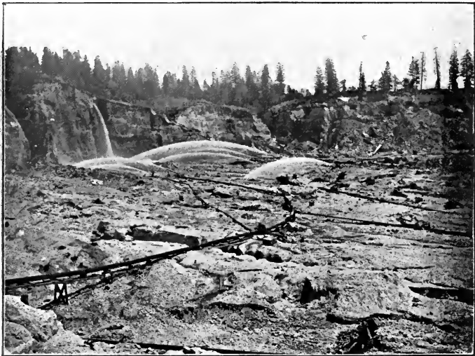
FIG. 139. — View in the Malakoff Hydraulic placer mine, North Bloomfield, California. From a photograph.
